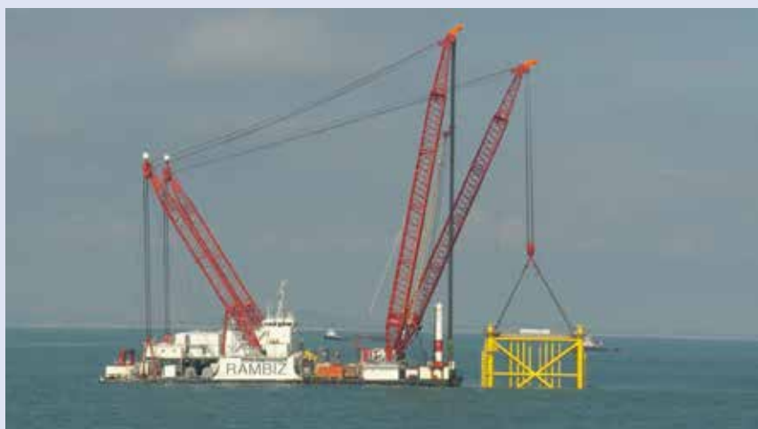
The jacket foundation for the offshore substation was installed last month
