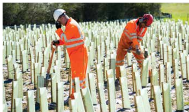
Trees are planted around the substation site
