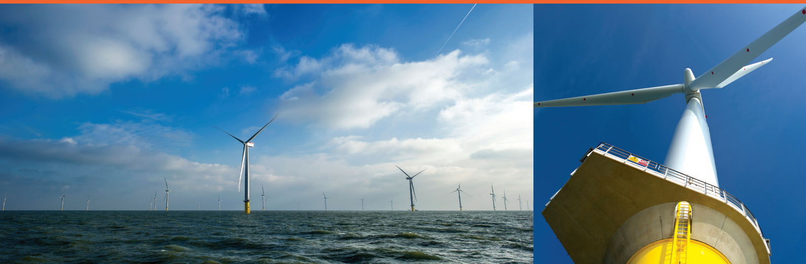
London Array Offshore Wind Farm. For illustrative purposes only.
