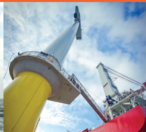
Final turbine installation, London Array, Thames Estuary.
