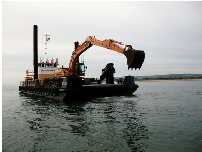
The Stour vessel with long reach excavator
